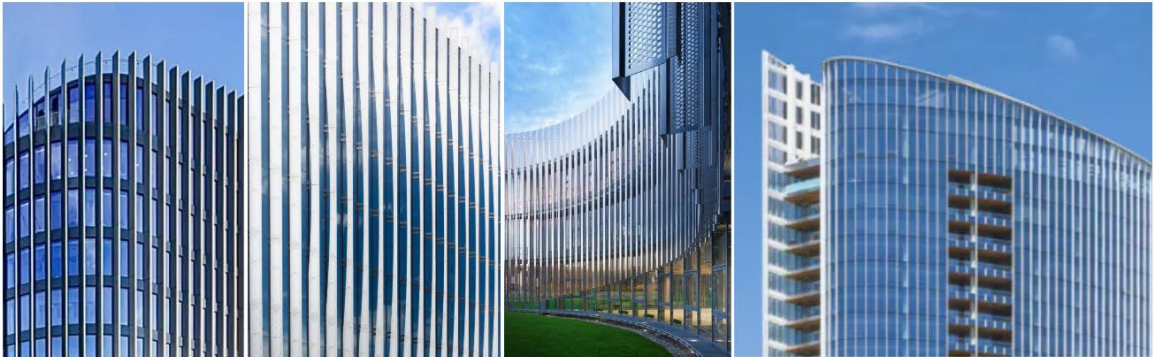
TRIPLE PANE GLAZING, METAL PANELS & FINS
