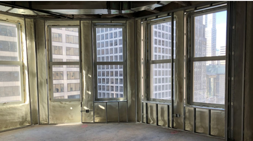
Historic facade receiving interior spray insulation (SCB). Hygrothermal analysis: Prudence.
