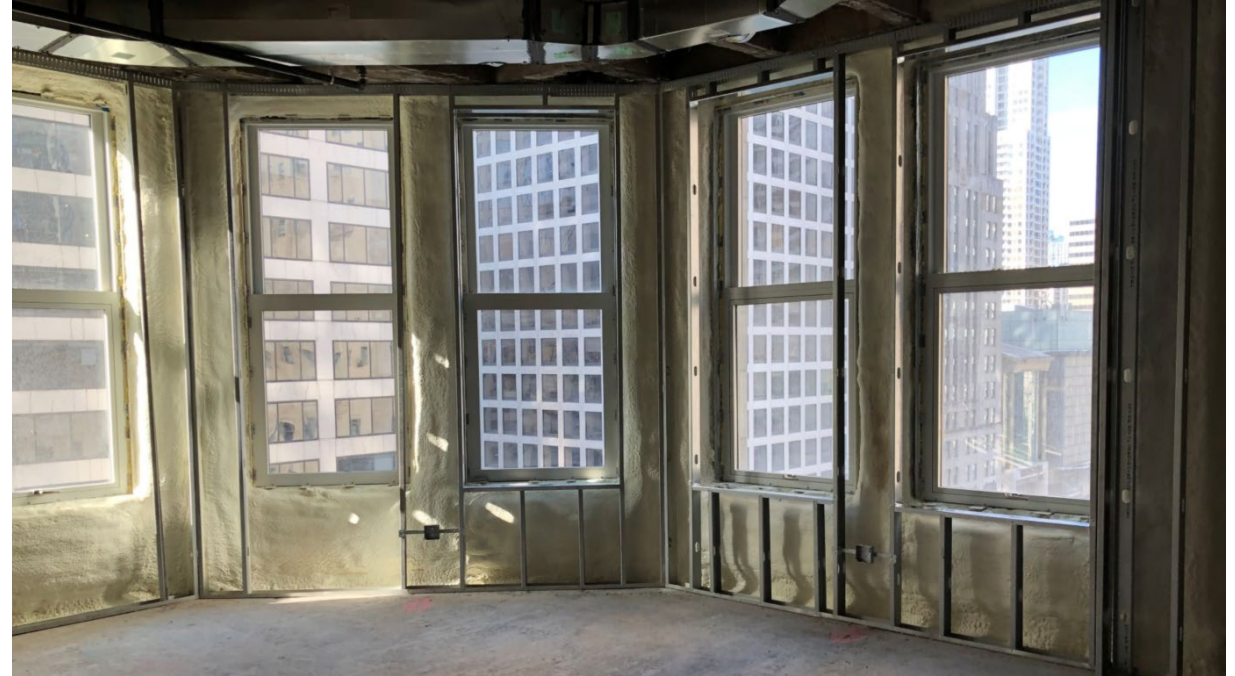
Tribune Tower (1930) – Receiving Spray Foam Insulation on the Interior
