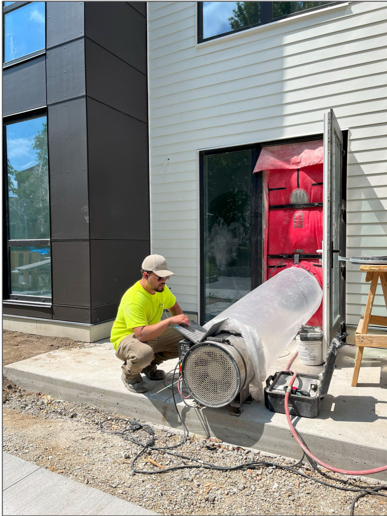
AeroBarrier Set Up Outside
