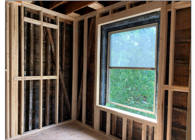
After New “Interior Wall” Framed
