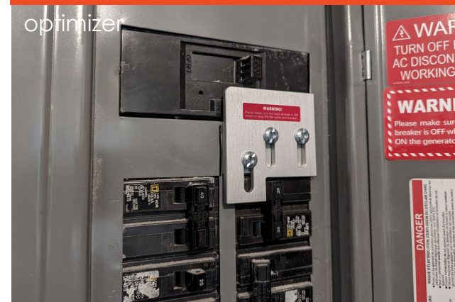
Interlock device for toggling power
