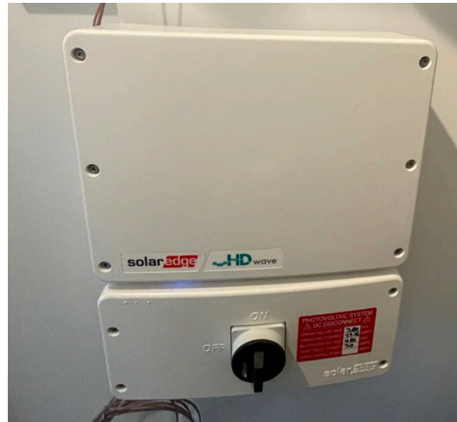
Solar Edge Inverter and power optimizer
