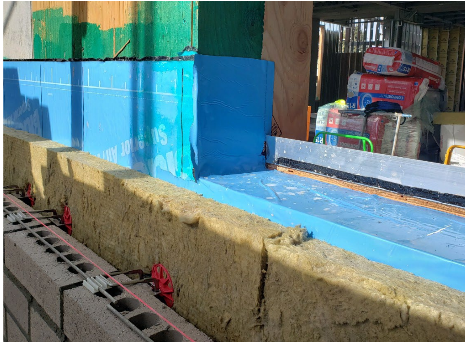
TYPICAL EXTERIOR PASSIVE HOUSE WALL (R-46.6)
