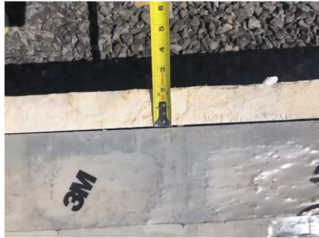
Do measure with measuring tape flat along insulation
