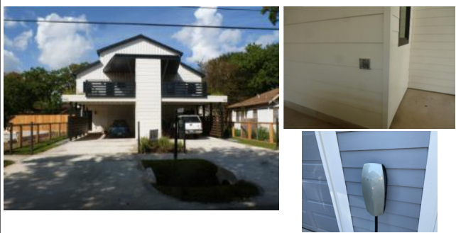
Do provide close photo of EV charging receptacle or charger.
