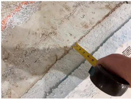
Don't measure with measuring tape at an angle.
