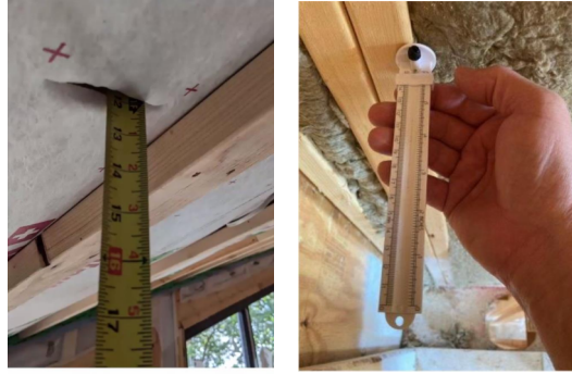
Do include photo that shows measured cavity insulation thickness.
