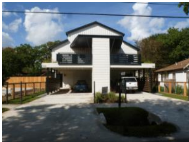
Don't take photo of EV charging receptacle from afar.
