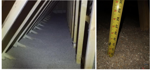
Do provide photo that shows ceiling insulation and measured insulation thickness.
