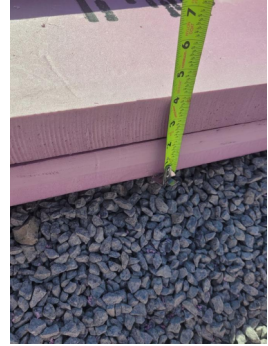
Do provide photo that shows context, measured insulation thickness, and manufacturer label.
