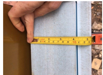
Do provide photo that shows context and measured insulation thickness.
