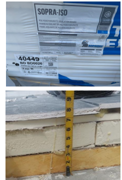
Do provide photo that shows context, measured insulation thickness, and manufacturer label.
