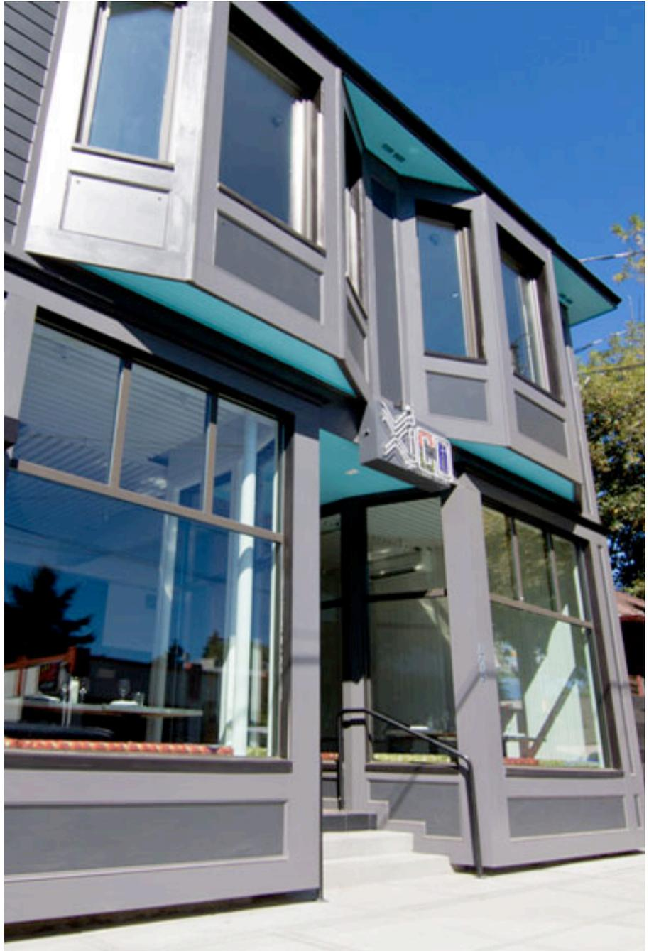
assembly the wall is R-33. The roof is an R-45 water-blown low density spray polyurethane (LDSPF) roof system with a sealed interior OSB air tightness layer.
