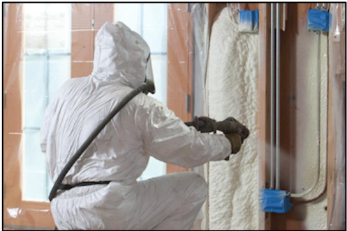
Spray Foam Insulation
