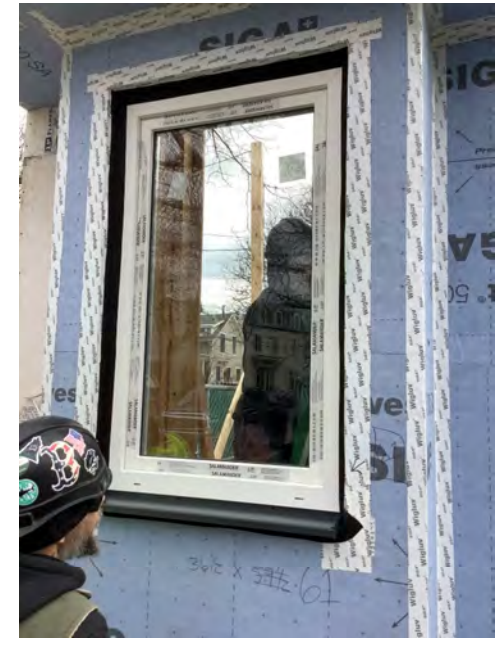
Leave up until installed in situ
