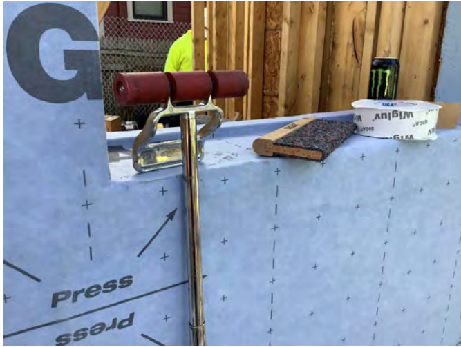
Require proper tools
