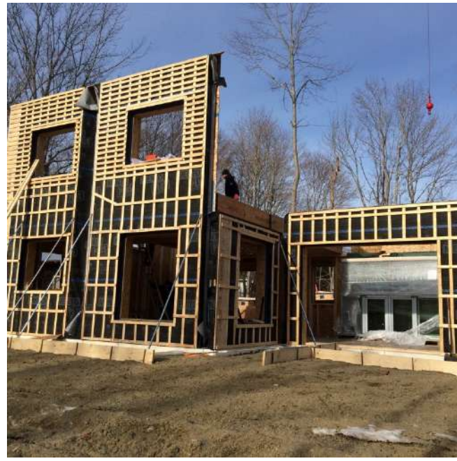
Above: wall section of Edgewaterhaus, Green design Studio, Double stud wall with air barrier on INTERIOR Right: Ecocor, prefabricated I-JOIST wall system for Gerard Haus.
