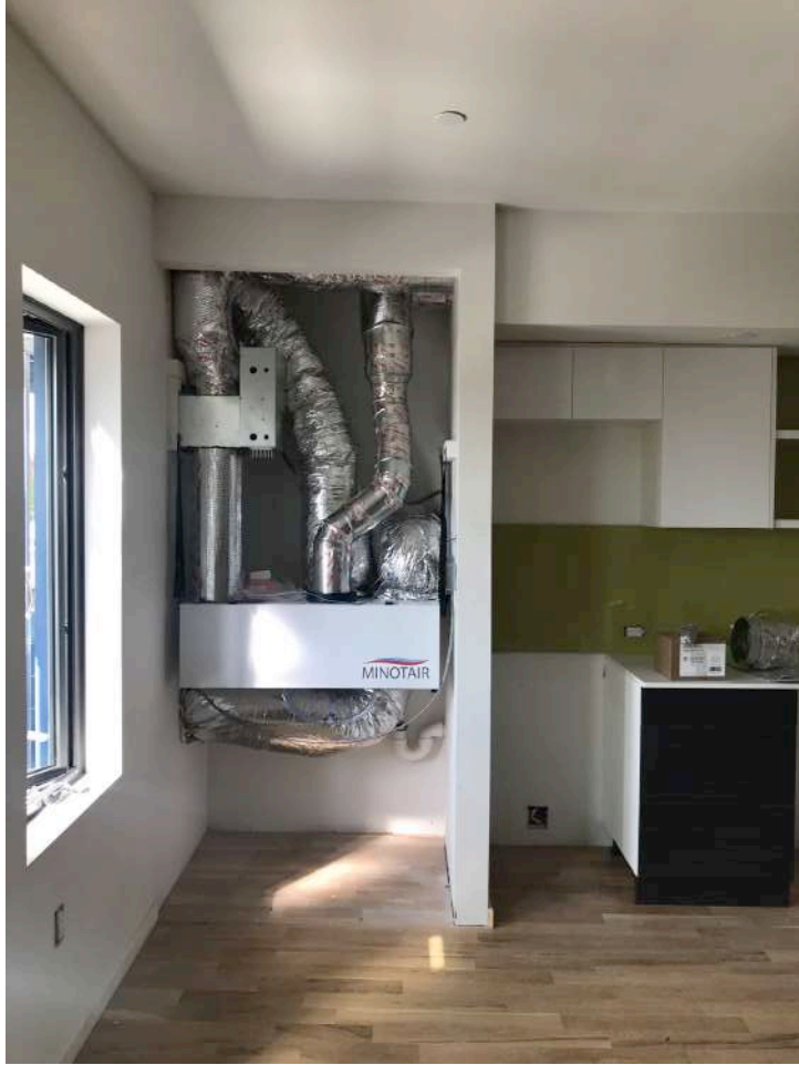
HVAC Closet merged with Kitchen cabinetry
