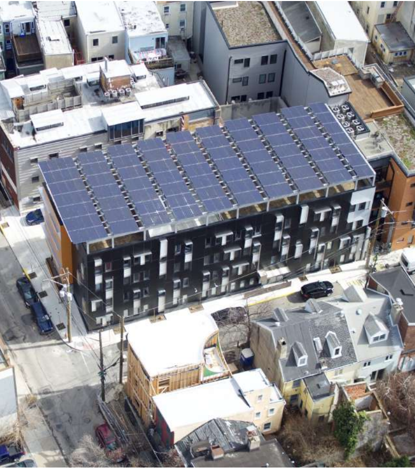
The Battery, PHIUS + Certified, 2017; 77 KW "BIFACIAL" PV ARRAY WITH ONE METER
