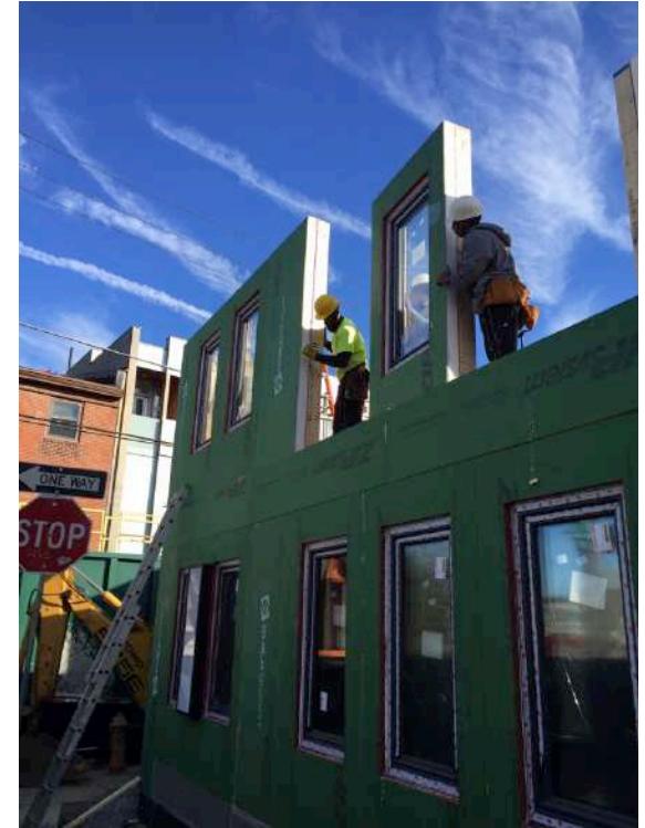
The Battery, PHIUS + Certified, 2017: Buildmart prefabricated wall system, windows/doors installed
