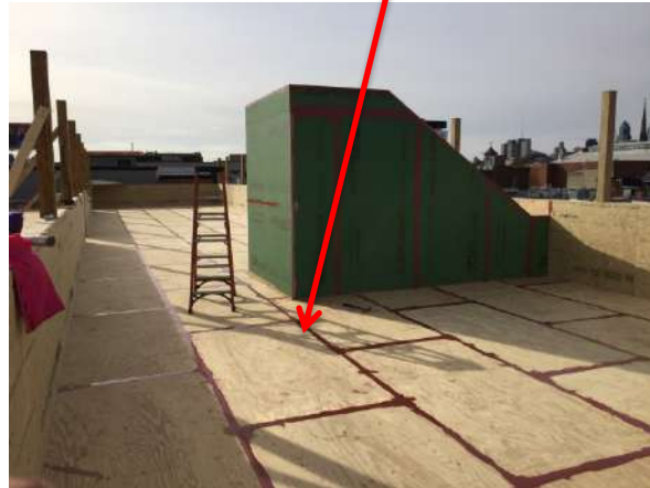
The Battery, PHIUS + Certified, 2017: FLAT ROOF, green roof, roof sheathing doubles as Air Barrier
