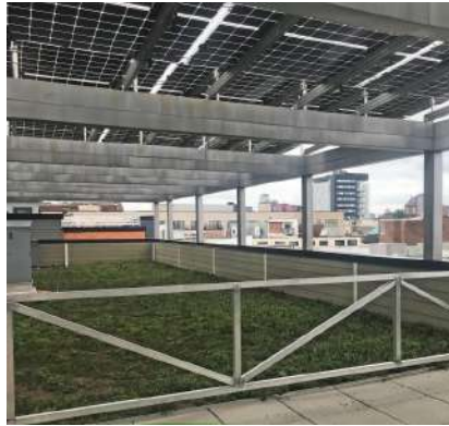
The Battery, PHIUS + Certified, 2017; 77 KW "BIFACIAL" PV ARRAY WITH ONE METER
