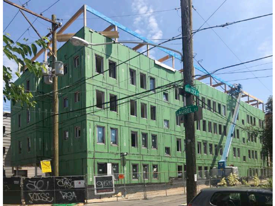
The Battery, PHIUS + Certified, 2017: Buildmart prefabricated wall system, windows/doors installed
