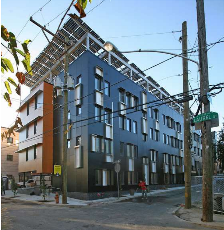
The Battery, PHIUS + Certified, 2017, OPEN LOOP, "STANDING COLUMN" GEO WELLS
