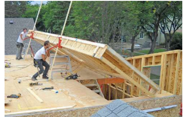
Above: wall section of Edgewaterhaus, Green design Studio, Double stud wall with air barrier on INTERIOR Right: Health Net Zero
