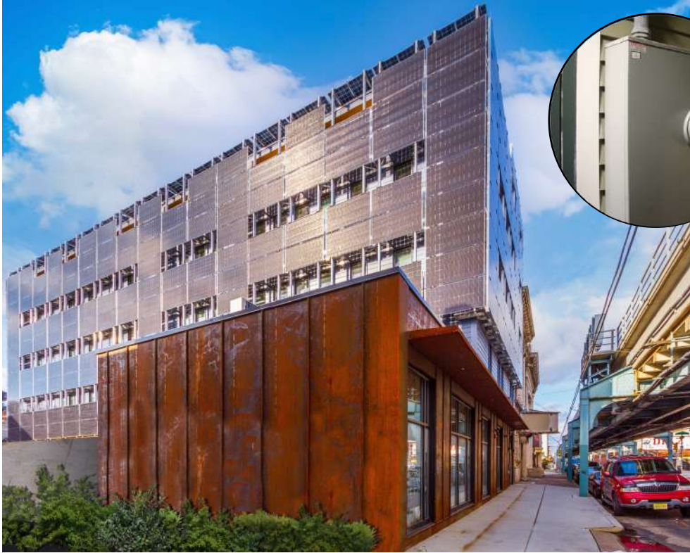
FRONT FLATS, 2019; 176 KW "BIFACIAL" PV ARRAY on façade AND ROOF WITH ONE METER
