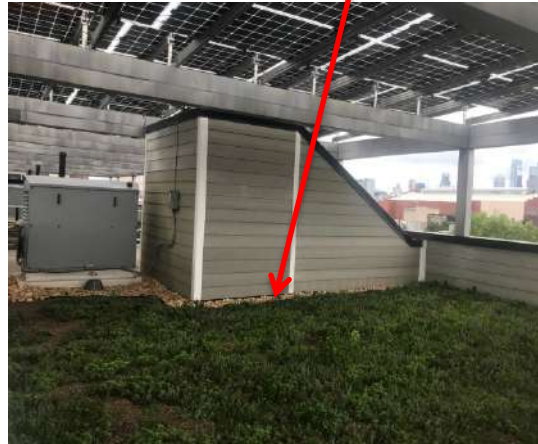
The Battery, PHIUS + Certified, 2017: FLAT ROOF, green roof, roof sheathing doubles as Air Barrier
